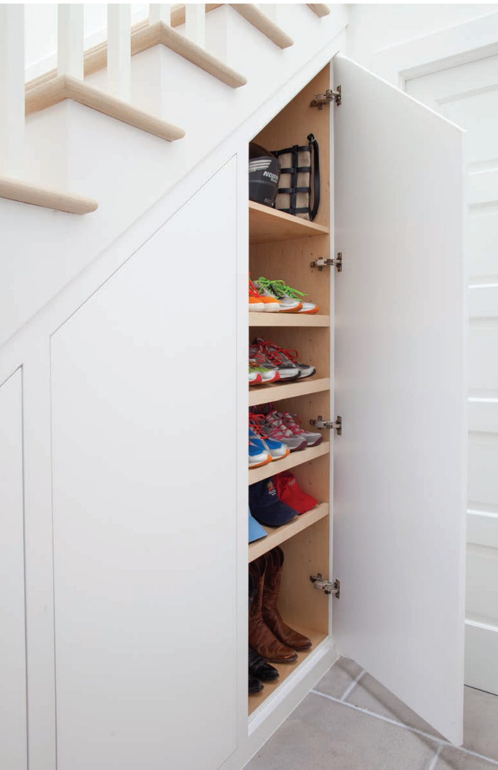
The new under-stair storage in the entryway holds quite a few pairs of colorful sneakers, Amy's beloved cowboy boots, and accessories for her spoiled pooch, Sadie. Amy liked the no-hardware look, so the Hemingway team installed touch latches to open the doors.
